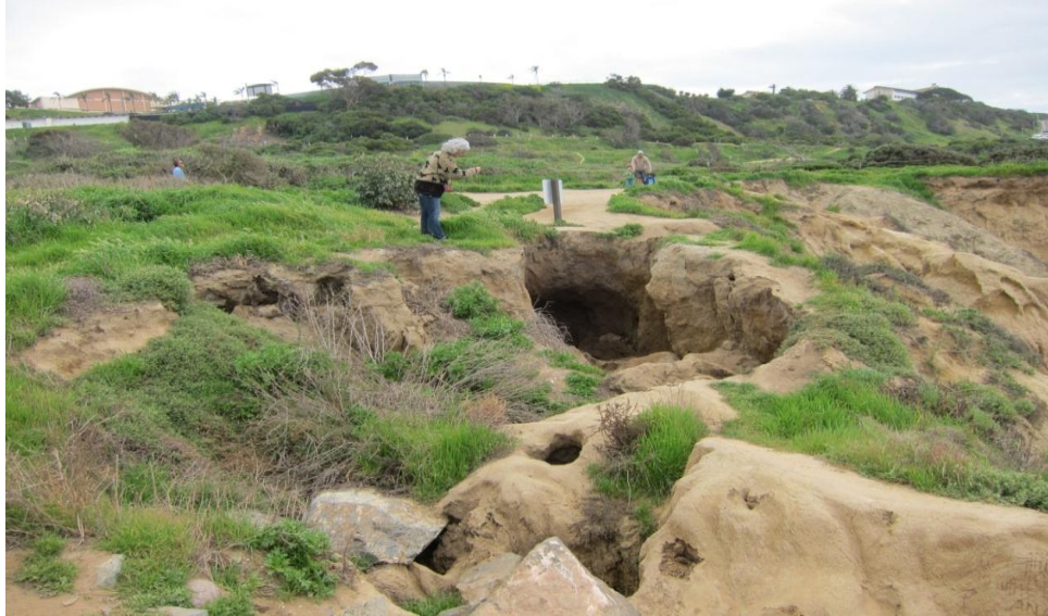
Figure 6. Erosion and sinkholes caused by runoff from the Lower Parking Lot.
