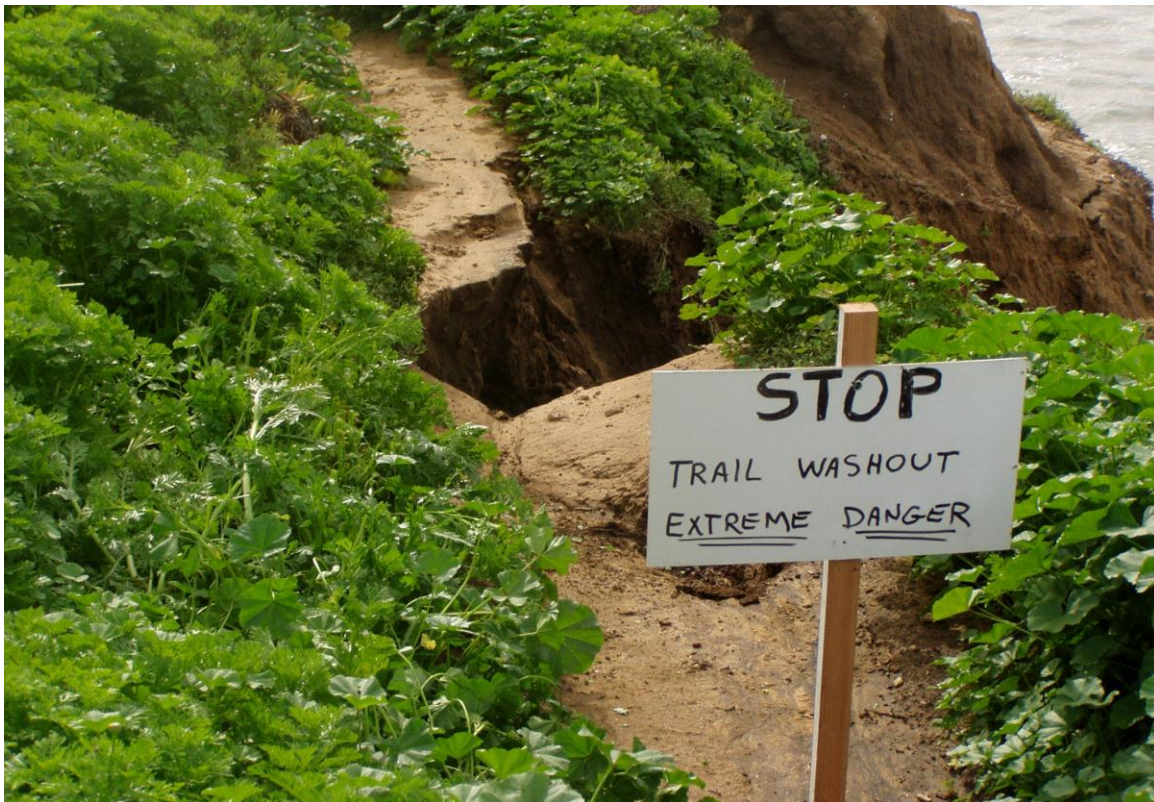
Figure 1. Erosion gully that in 2005 severed the main trail along the cliff from the Ladera and Sunset Cliffs corner to the Lower Parking Lot
